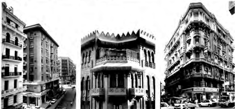
Prominent buildings in Cairo’s city center built during the belle époque (photographs by Alain Bonnamy).
