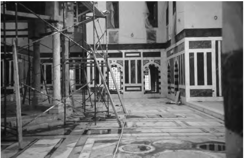
Madrasa of Sarghatmish (1356) the interior courtyard, with new marble contrasting with original marble floors and walls (photograph by Caroline Williams).
