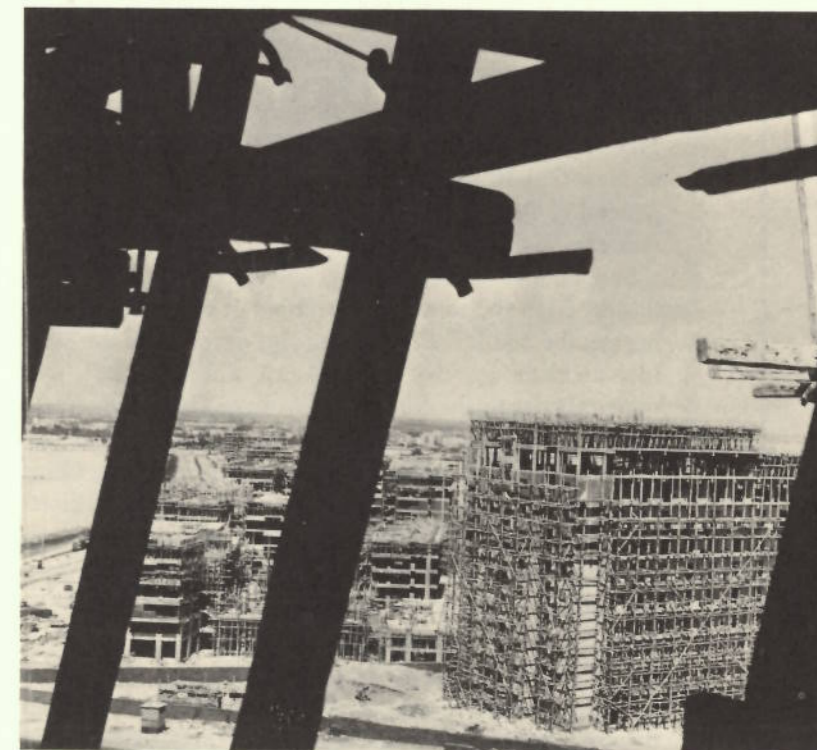
156. Naṣr City, still under construction
