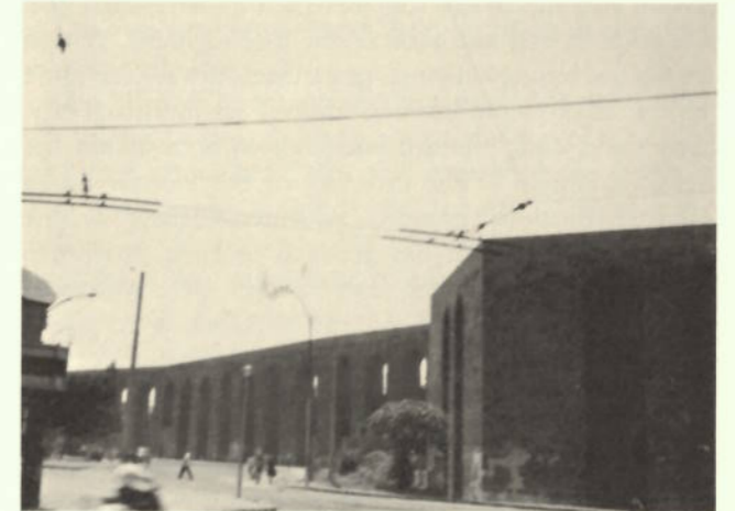
37. The aqueduct today, surrounded and functionless
