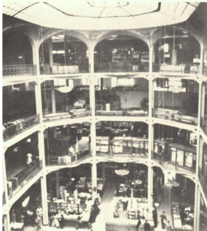
One of Cairo's earliest "new style" department stores: Sednoui's
