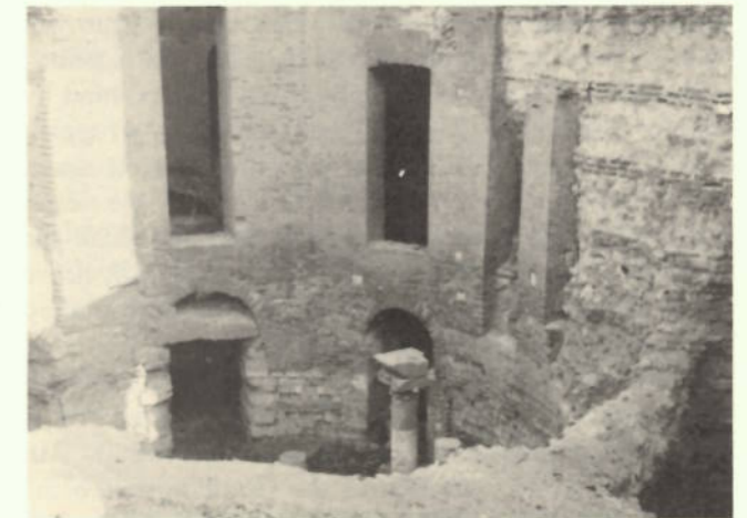
4. Fortress now far below ground level
