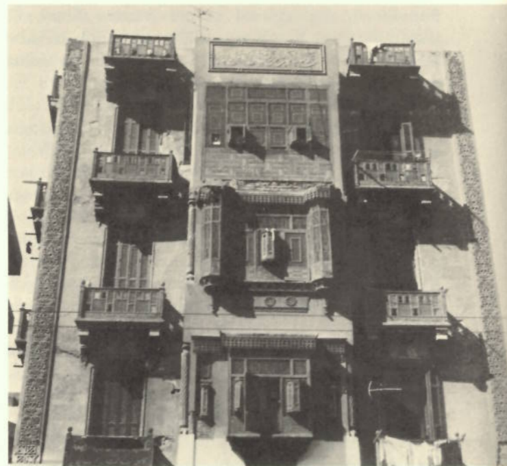
52. Windows and balconies of a house in Būlāq
