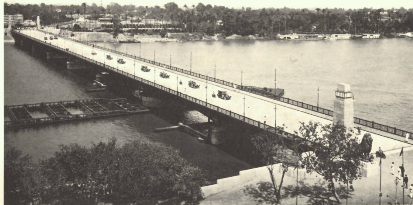
68. Second Qaṣr al-Nīl Bridge
