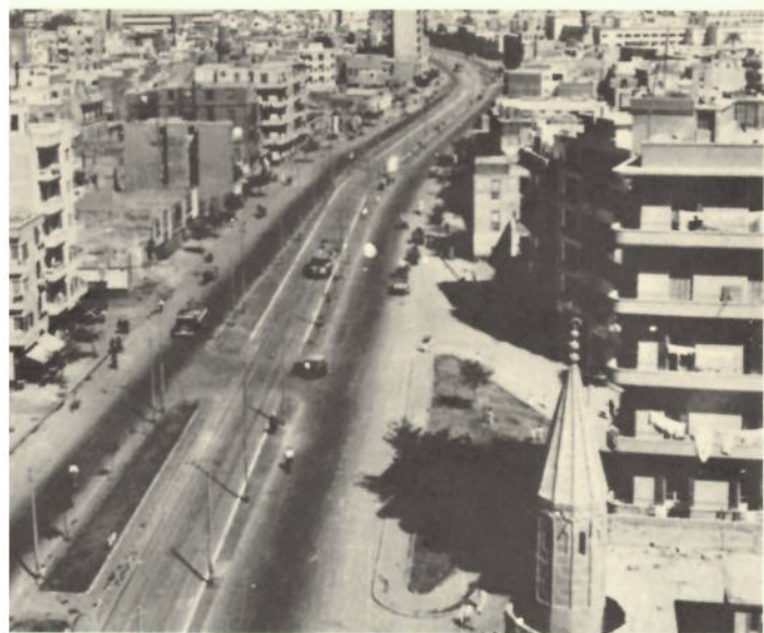
76. Port Sa'id Street, today's widened thoroughfare, follows the old bed of the Khalij canal and street
