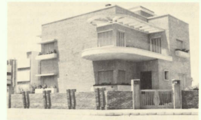
140. The other side of the street: new villa of Maḍīnat al-Muhandisīn, 1965
