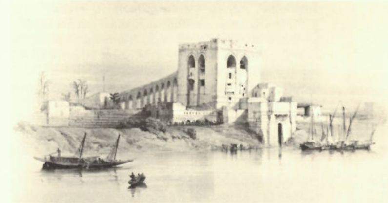
36. Unchanged landmark: al-Ghūri aqueduct near Fam al-Khalij ca. 1840
