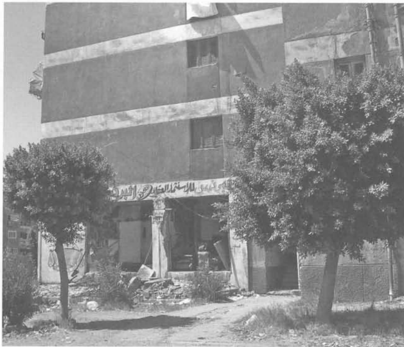
Figure 5.4. Demolished ground-floor shop in public housing in Sixth of October. (Photograph by Sonja Spruit.)
