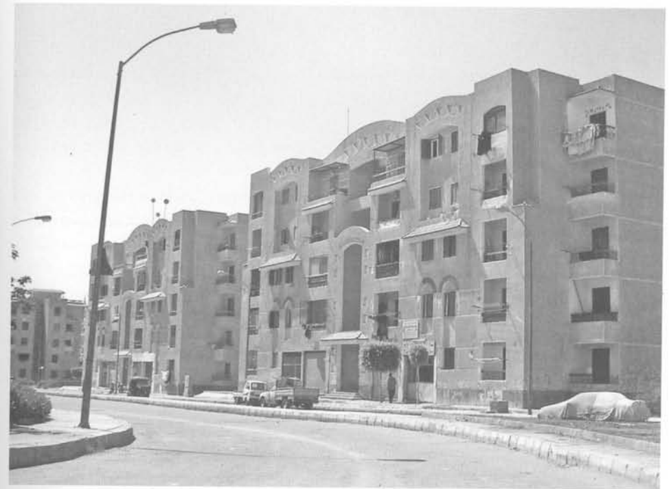
Figure 5.5. Example of Mubarak Youth Housing in Sixth of October, built 1997–2000. (Photograph by Sonja Spruit.)
