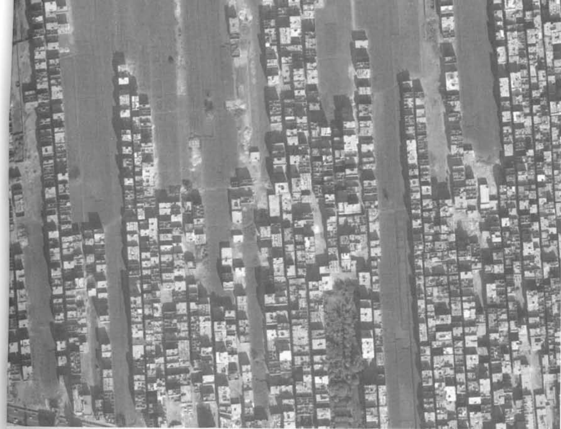
Figure 4.11. Informal development by converted agricultural strips in al-Bashtil, Giza. (Image dated 2008, ©2010 DigitalGlobe / ©2009 GOOGLE.)
