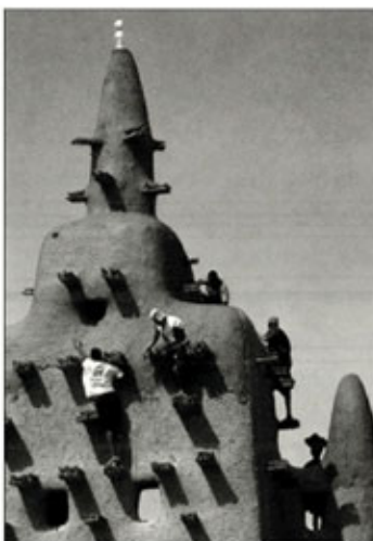
Great Mosque at Djenne, Mali. Men resurfacing mihrab tower.
