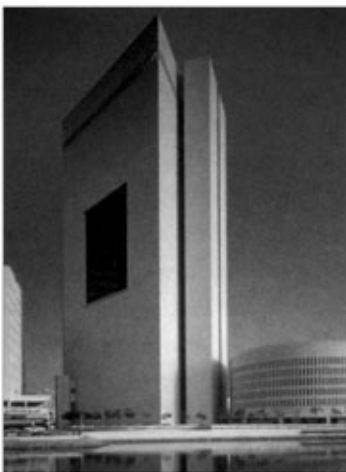
Modern versions of the tall building must also be suited to the environment. SOM’s dramatic National Commercial Bank building in Jeddah, Saudi Arabia, deals effectively with sun and glare.
