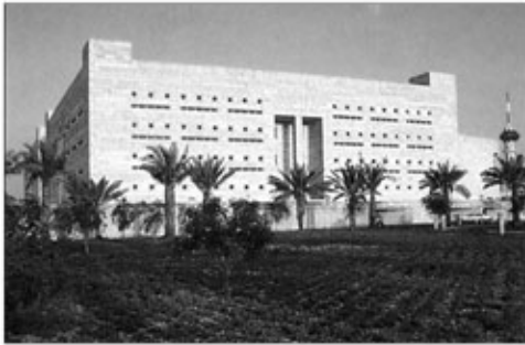
Henning Larsen, Ministry of Foreign Affairs, Riyadh, 1984 . The fortress-like protected outside wall defines intricately detailed interiors.
