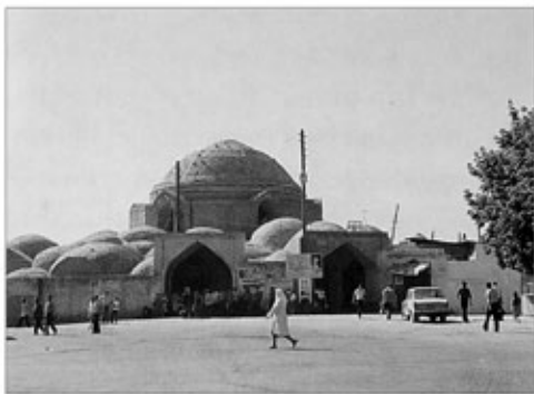
Bukhara, remains of sixteenth century bazaar.
