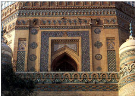
Two approaches to restoration: Externally the old and the new are clearly distinguished as in Darb Qirmiz, Cairo (top) or are indistinguishable, but are clearly labelled in unseen areas as in Multan, Pakistan (above).
