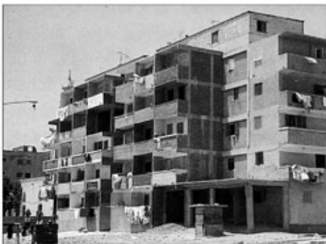
Unregulated expansion of apartments in public housing blocks.
