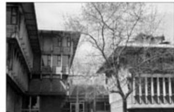
The Social Security Complex Istanbul, Turkey, completed 1970 1986 winner
