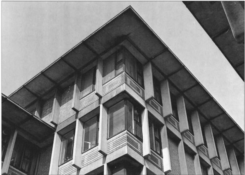
Above: Elevation showing treatment of vertical louvres and cement tiles. Right: The purity of the angular connections can be seen at the different levels of interconnection.
