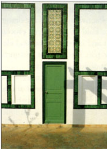
The open courtyard and the use of water in Résidence Andalous (top) give it a distinctly local flavour, even though decorative elements were used sparingly and in modern abstract designs (above).
