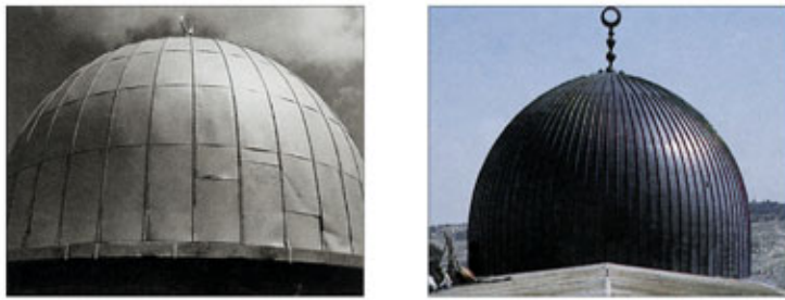
Exterior of dome before and after restoration.
