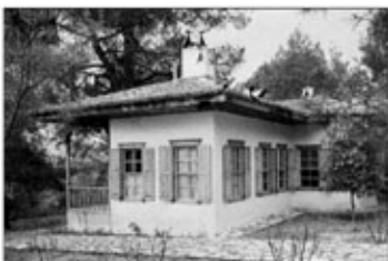
Nail Çakirhan Residence Akyaka Yillage, Turkey, completed 1971 1983 winner
