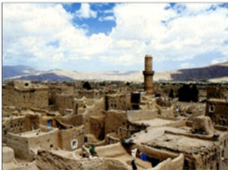
View of Amran, Yemen. Architecture, whether done by the medium of architects or only builders, is by necessity a physical mirror of a society's social, economic, cultural, legal and technological realities as well as an adaptation to the physical environment.
