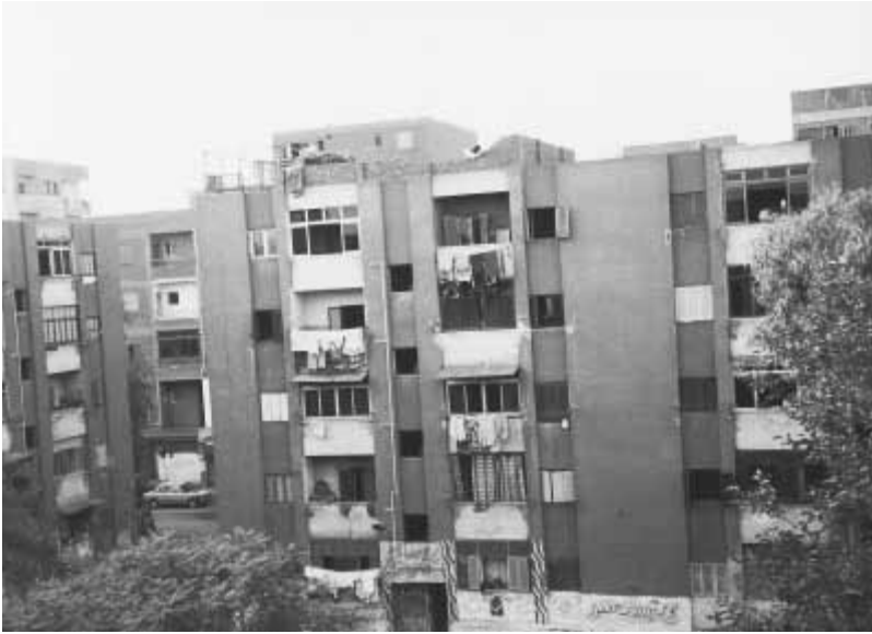
FIGURE 6: The original design of the balcony can be seen on the second and fourth floors (the left side of the photograph). The most expensive alterations are on the third and fifth floors. Notice that to ensure visual protection, balconies on the ground floor are covered with wooden shutters. Photograph by Farha Ghannam.
